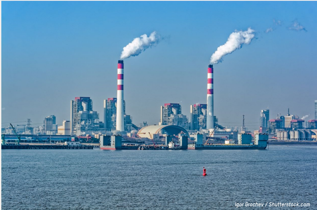
View of the largest coal-fired power plant in China (Shanghai).
